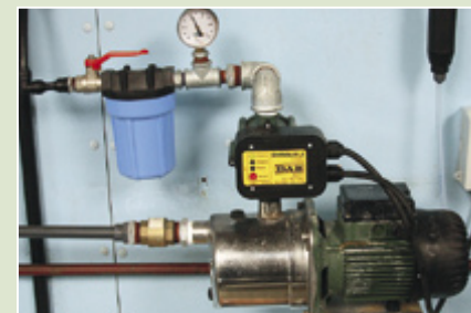
The heart of the AirWash system is the pump that, on demand, takes the fluid to the parlour-based controller and then, when required, on to the clusters.
