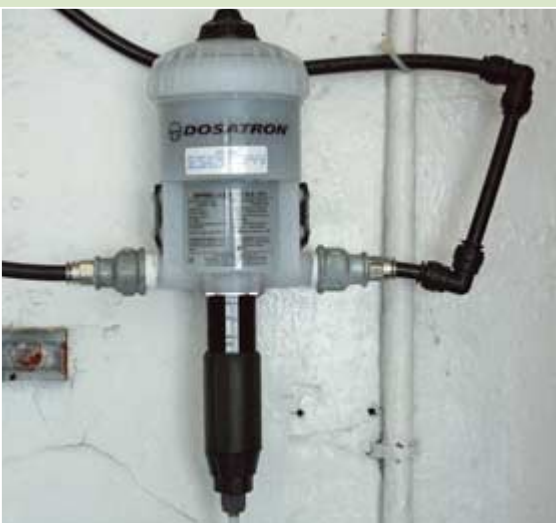
Peracetic acid is metered out by this dosing system. The concentration can be adjusted to suit.
