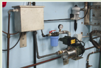
Peracetic acid is added to the flushing system header tank – to maintain the required solution. The dosing unit can be seen attached to the pipe on the right.
